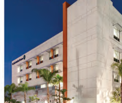
St. Jude Medical Center Northwest Tower
