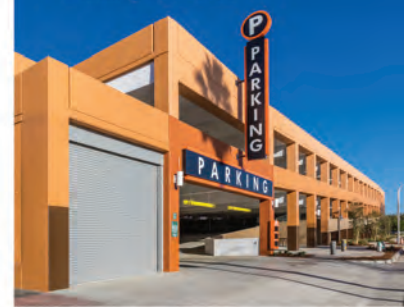
Brea Superblock I Parking Structure
