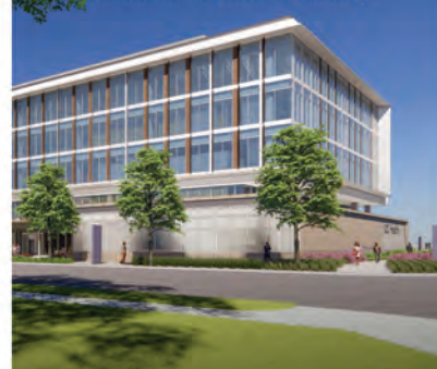
UCI Center for Advanced Care Medical Office Building
