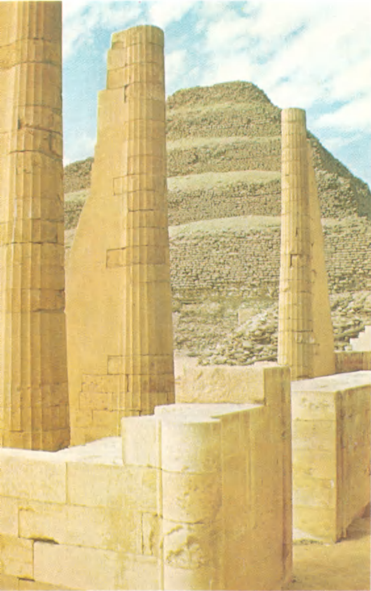
DJOSER'S TEMPLE and step pyramid (background) at Sakkarah, although the first all-stone structures, were nevertheless built along lines used by architects accustomed to working with mud bricks.
